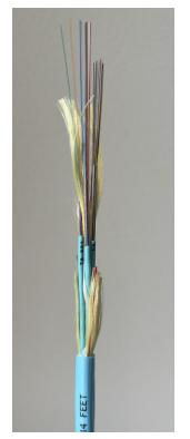
Manchester, NH – July 25, 2024—Proterial Cable America (PCA) has announced the release of **NanoCore® Micro Distribution** cables, which are **Base-8 and Base-16 fiber optic cables** ideal for use in hyperscale data centers due to their ability to efficiently carry large amounts of data at high speeds.
